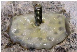
**7** Cure time varies with temperature. Surface and room temperature should be above 55°F/12°C. Allow to cure before applying load (approximately 30 min. at 70°F/21°C).
