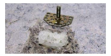
Place the fastener into the adhesive and apply pressure until adhesive is forced through the holes.
