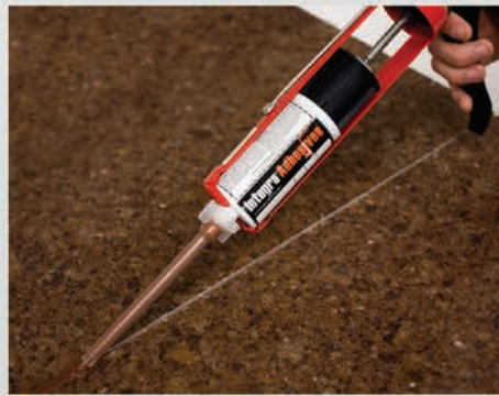
Deck Seams and Installations
